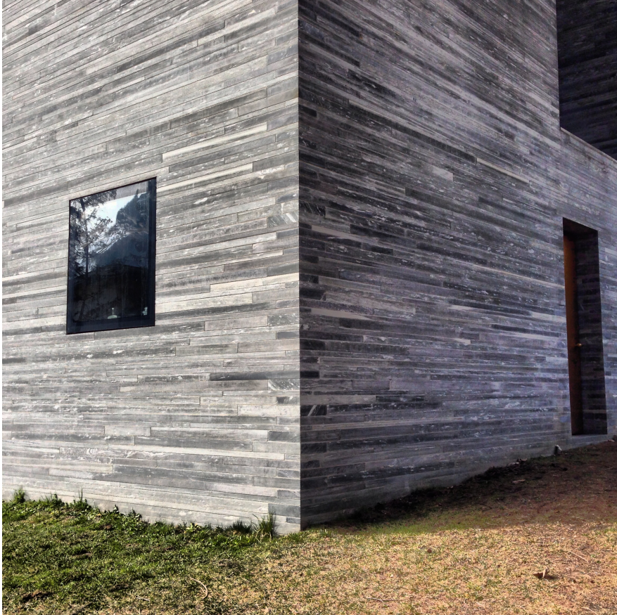
Figure 4.1: Detail of the Stonework in the Therme Vals hotel building by Peter Zumthor - photo credit: Marco Palma.
